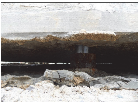
Figure 8. The Image Which is 100mm Lifted up
